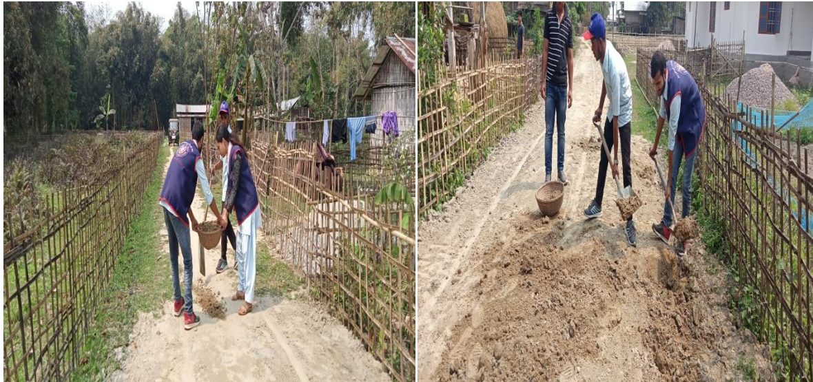
NSS Volunteer repairing Road & Cleaning the Campus
