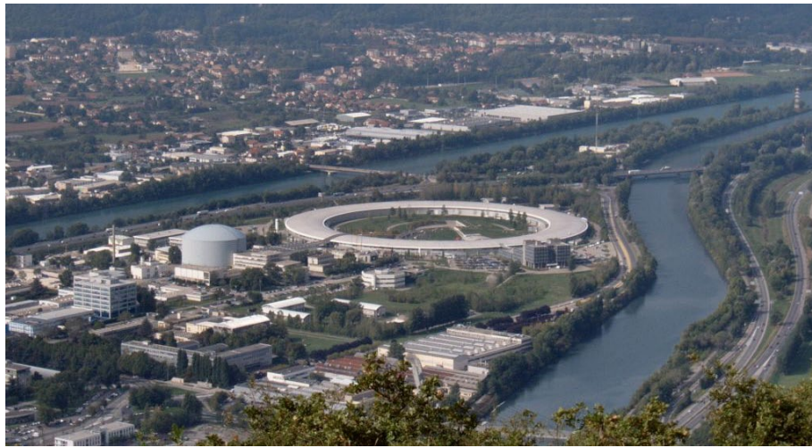
The European Synchrotron Radiation Facility in Grenoble, France. A synchrotron light source uses electrons accelerated to almost the speed of light in a giant storage ring to produce very bright X-rays. The ring is hundreds of meters in circumference; it can take 15 min to walk around the facility.
